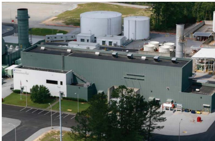
Figure 3. The McIntosh CAES Plant (Source: DOE Global Energy Storage Database)
