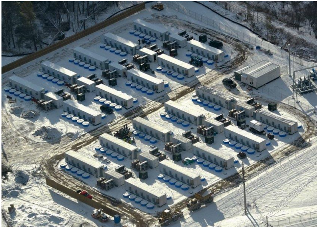
Figure 4. Beacon Power's flywheel energy storage plant in Stephentown, New York. (Source: Beacon Power)
